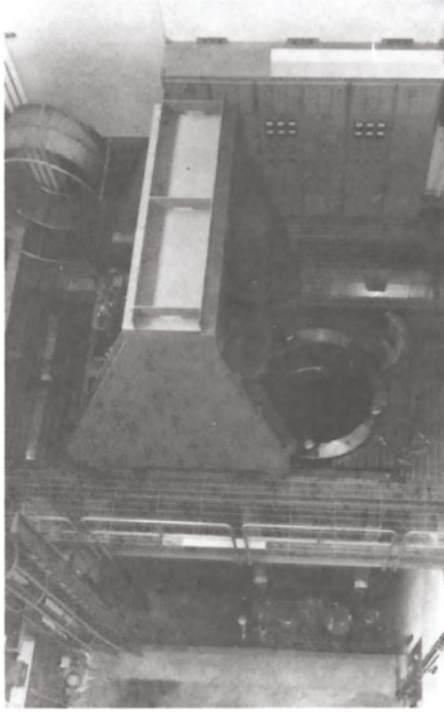
Figure 34. The large HIP vessel, as installed at Battelle, to be transferred to the Crucible Compaction Metals Operation. (Courtesy of Crucible Steel)
